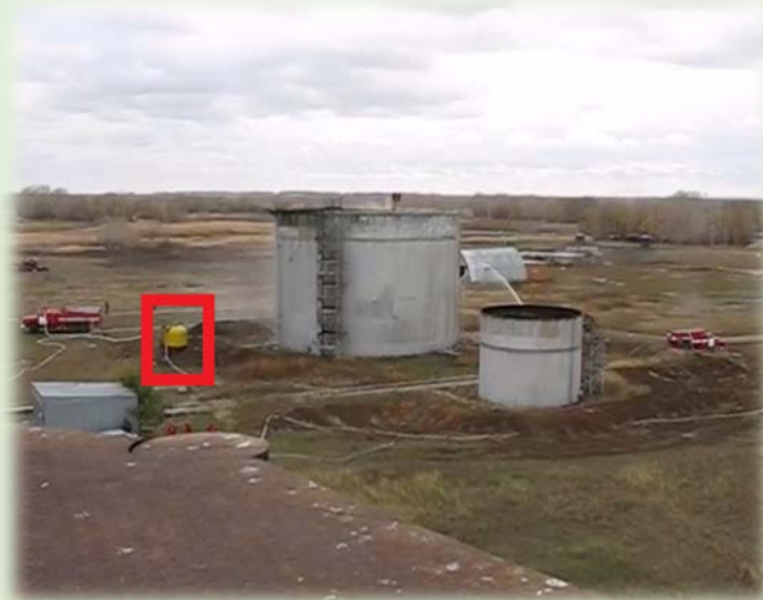
Just one device Isa-7500 extinguishing fire oil tank for 5 000 tons.
